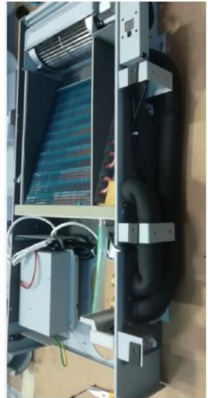
PUT INSULATION IN ALL THE EXTERNAL PIPE
