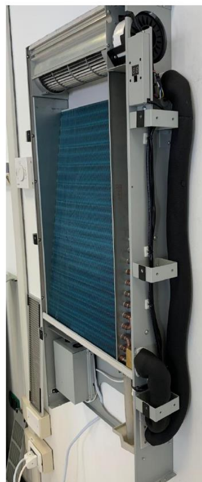
PUT INSULATION IN ALL THE EXTERNAL PIPE
