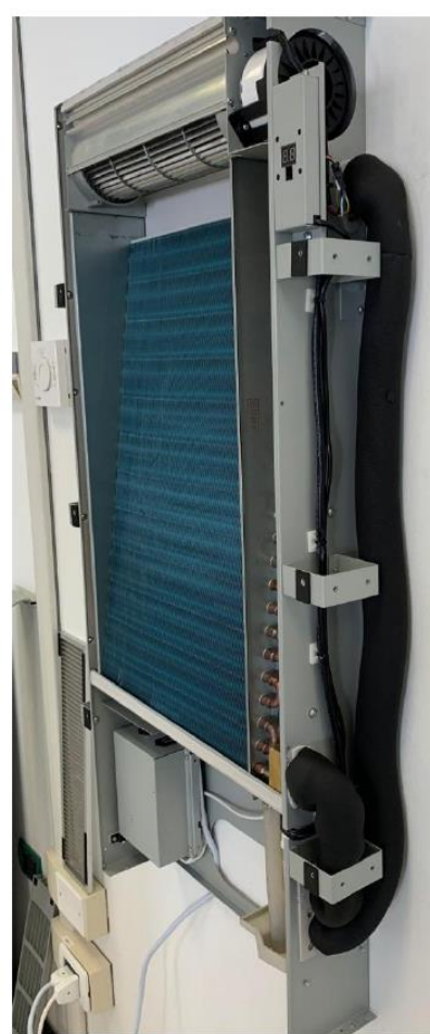
PUT INSULATION IN ALL THE EXTERNAL PIPE
